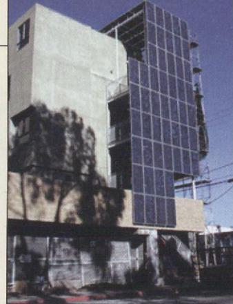
Santa Monica Green Building Program
