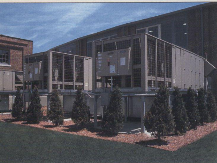
Renovation of the Kansas City-based DST Systems, Inc. property included the installation of energy-efficient York rooftop HVAC units.
