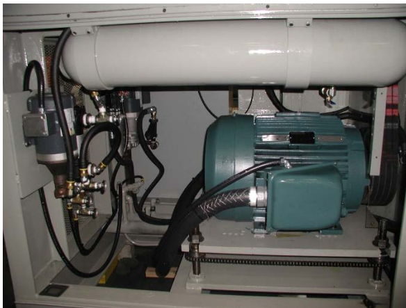
Variable Frequency Drive Retrofit
