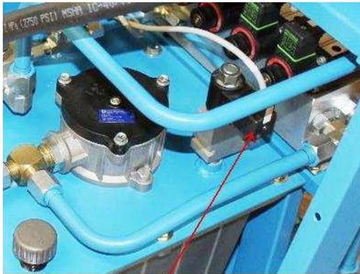
ACCUMULATOR DUMP VALVE CONTROL CABLE
