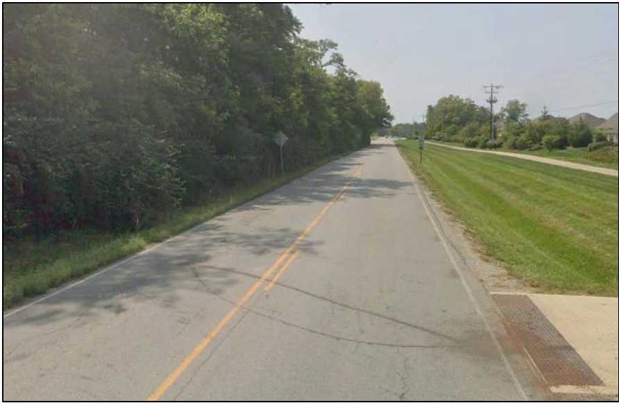
West Leg – Looking West
