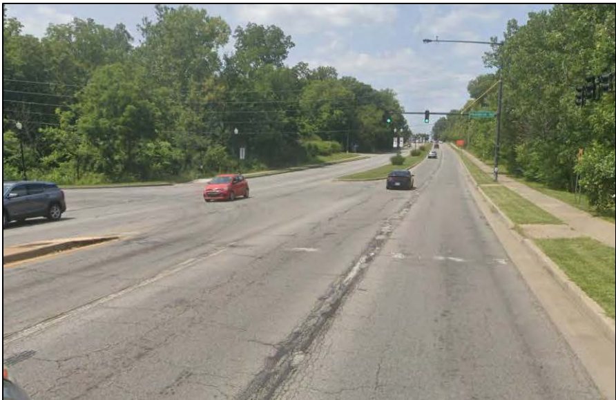
East Leg – Looking West
