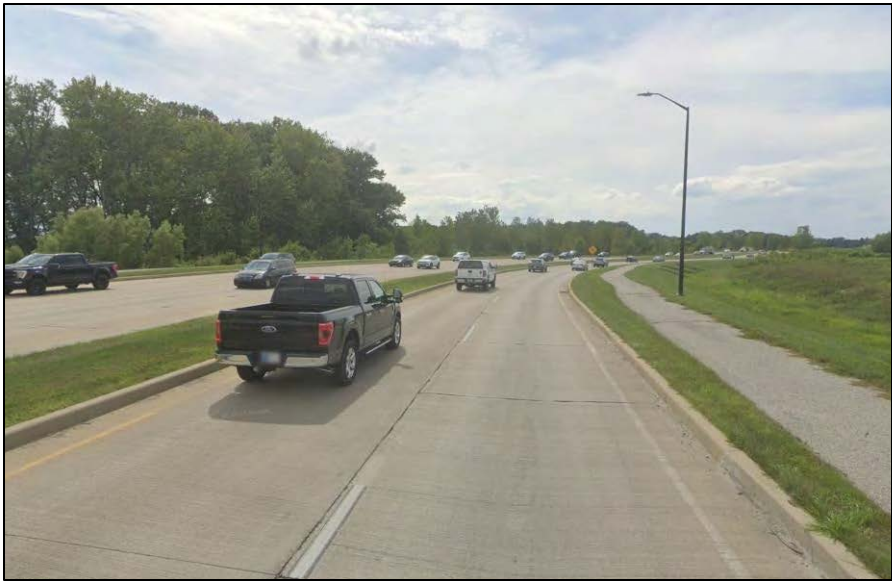
West Leg – Looking West
