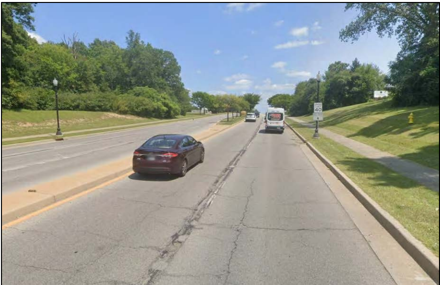
East Leg – Looking East
