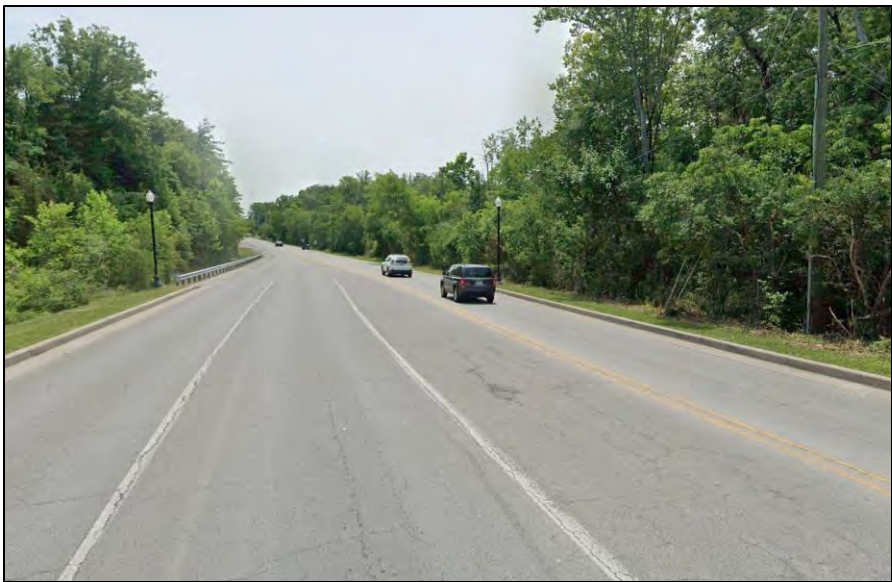
South Leg – Looking South
