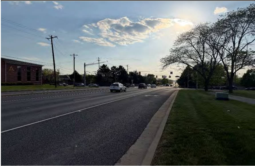
East Leg – Looking West
