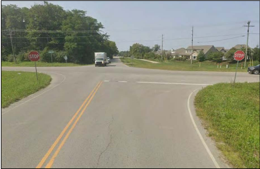
East Leg – Looking West
