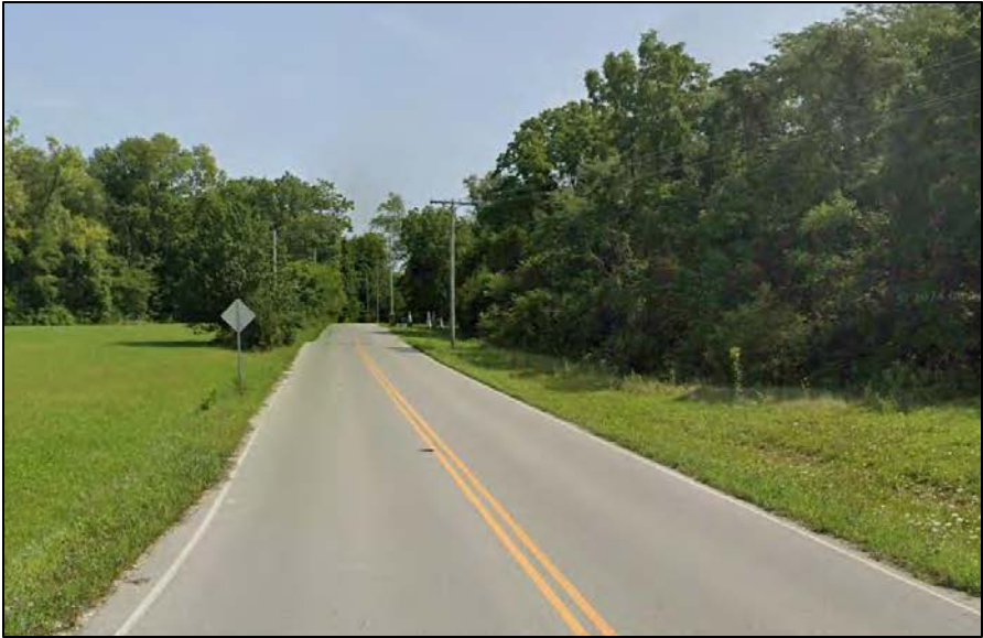
East Leg – Looking East
