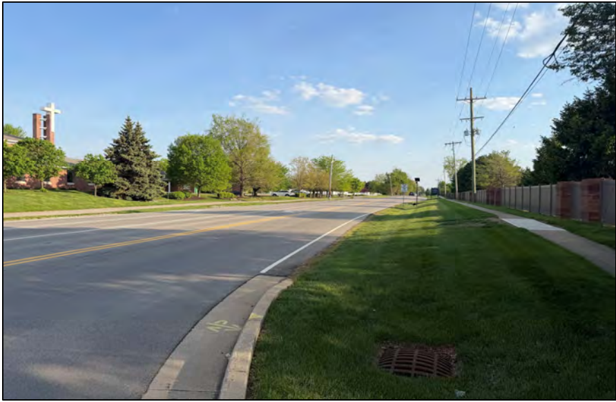
South Leg – Looking South
