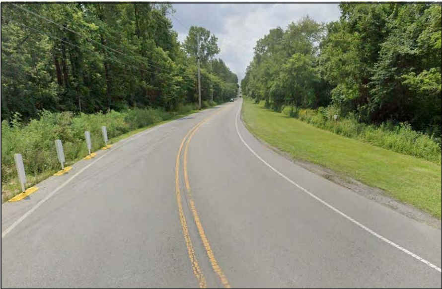
South Leg – Looking South
