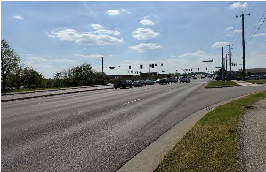
East Leg – Looking West
