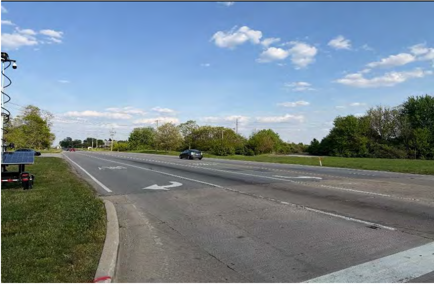
East Leg – Looking East
