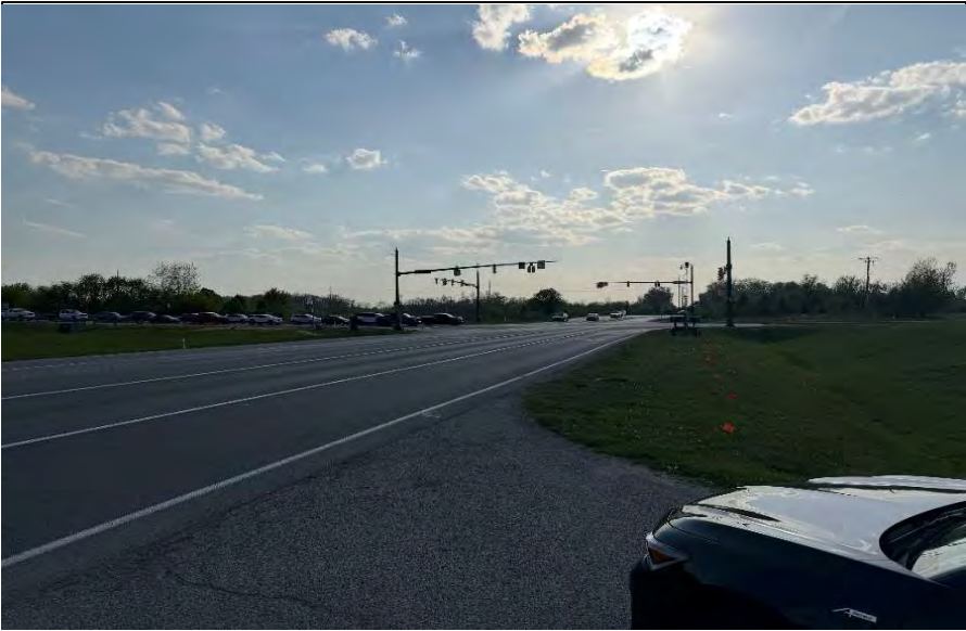
East Leg – Looking West
