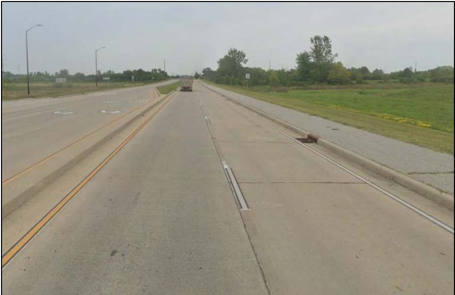
North Leg – Looking North
