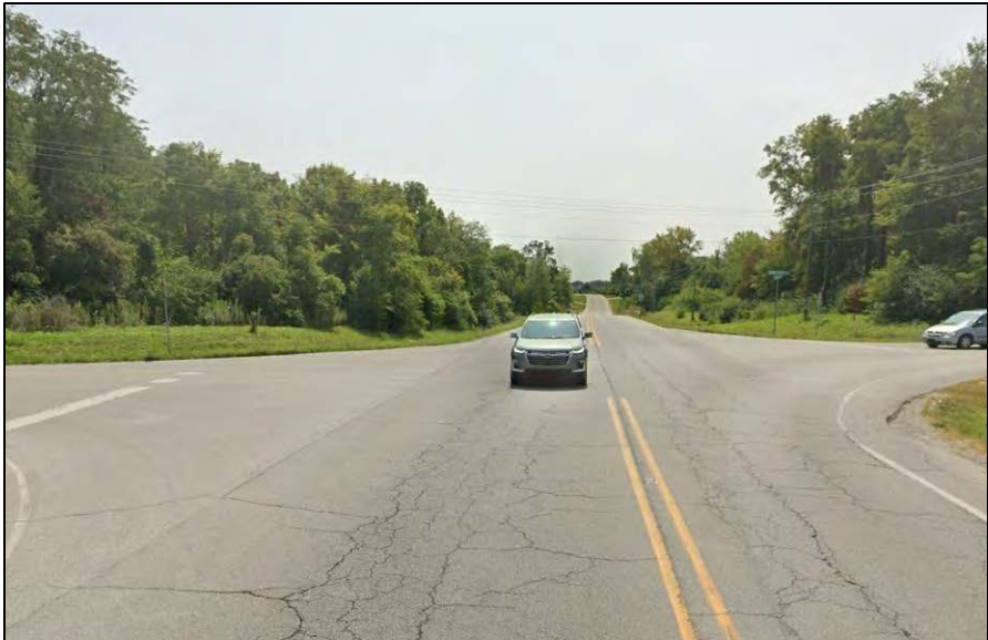
North Leg – Looking South
