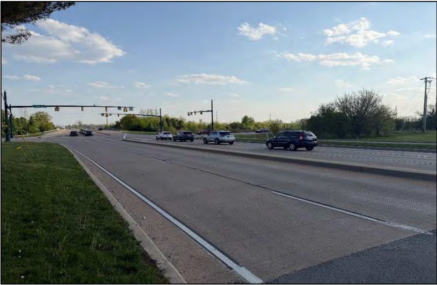
North Leg – Looking South
