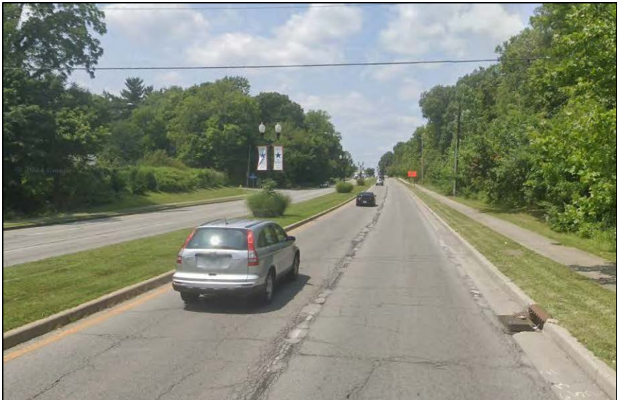
West Leg – Looking West
