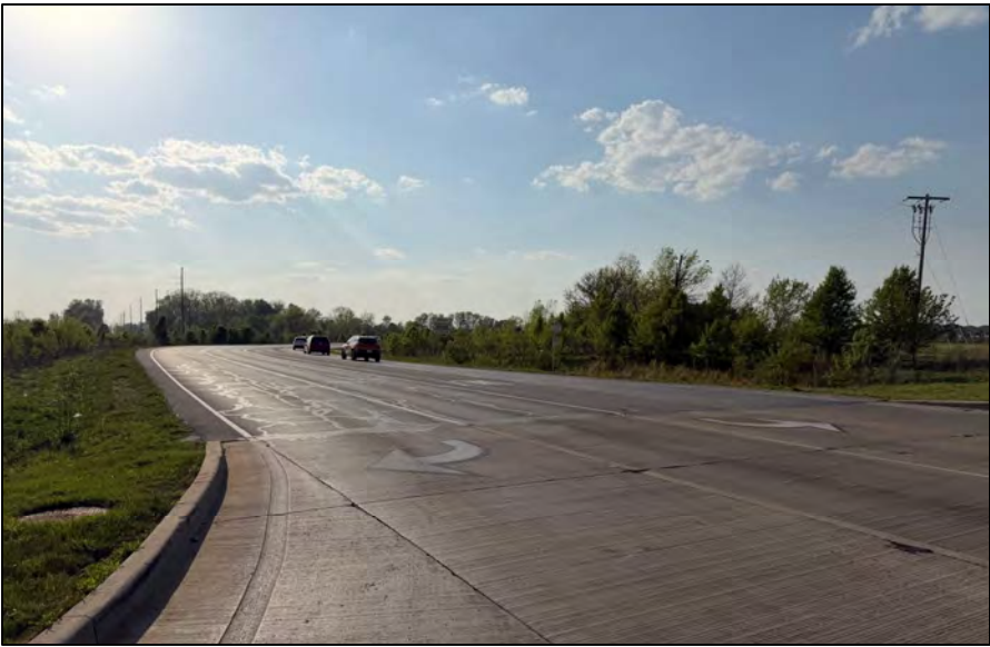
West Leg – Looking West
