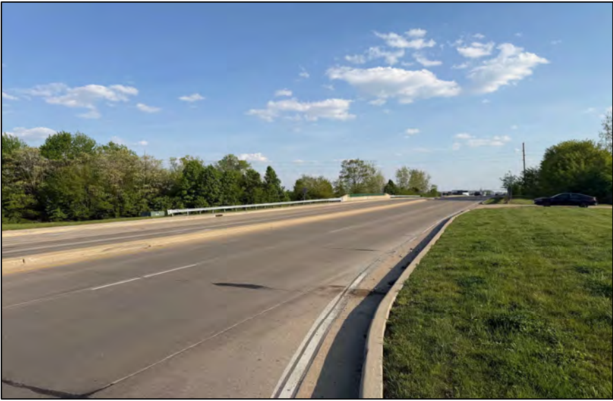
South Leg – Looking South
