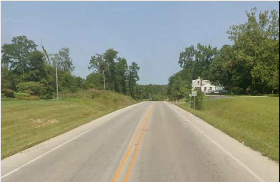
North Leg – Looking North
