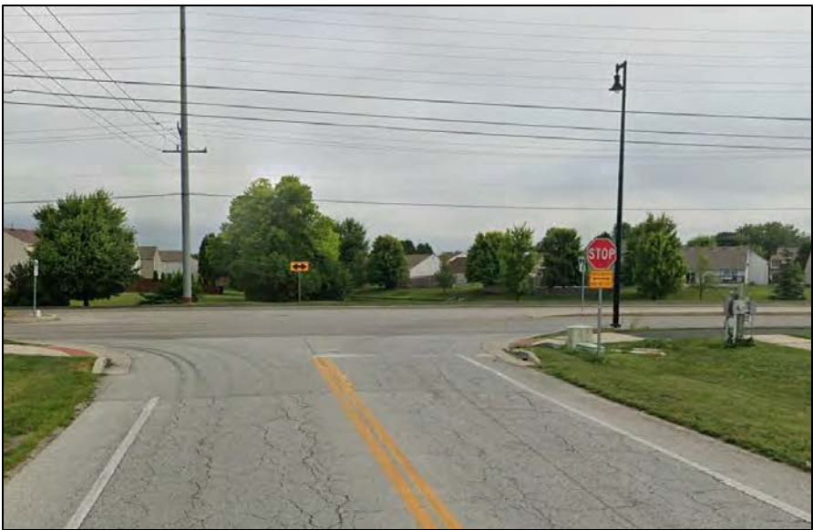
South Leg – Looking North
