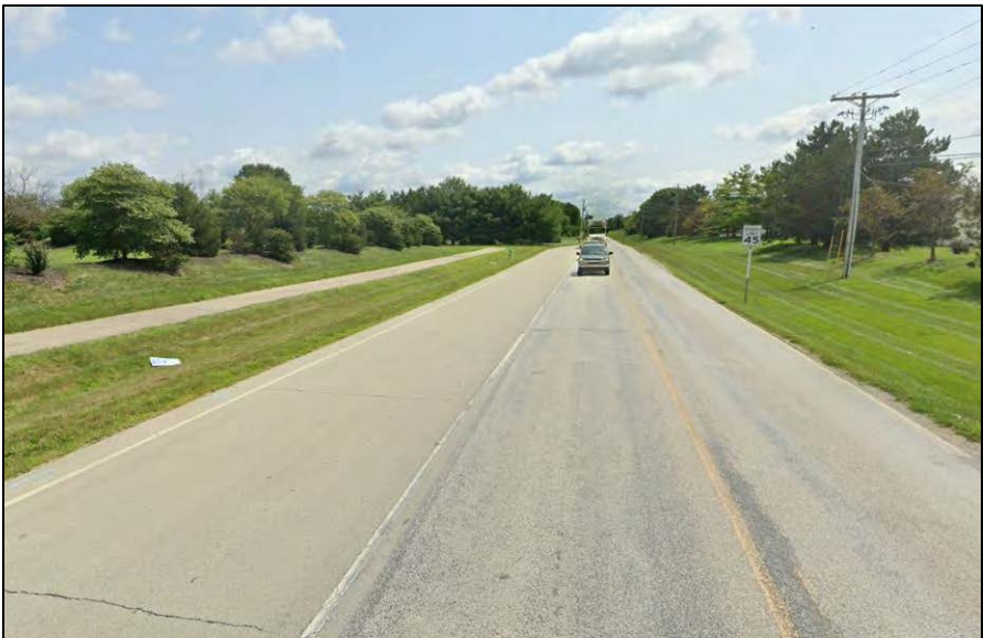
East Leg – Looking East
