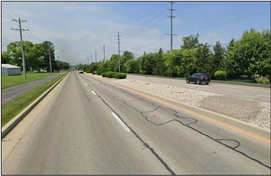
West Leg – Looking West
