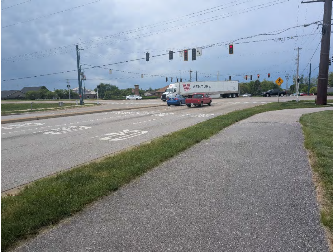
1. Looking west at east approach
