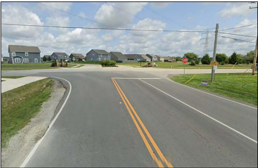
South Leg – Looking North
